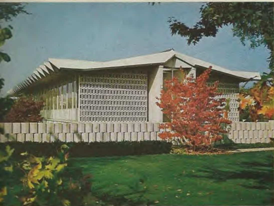
CONCRETE SHOW PLACE for American Concrete Institute uses concrete from roof to grille. Precast roof was lifted in place.
