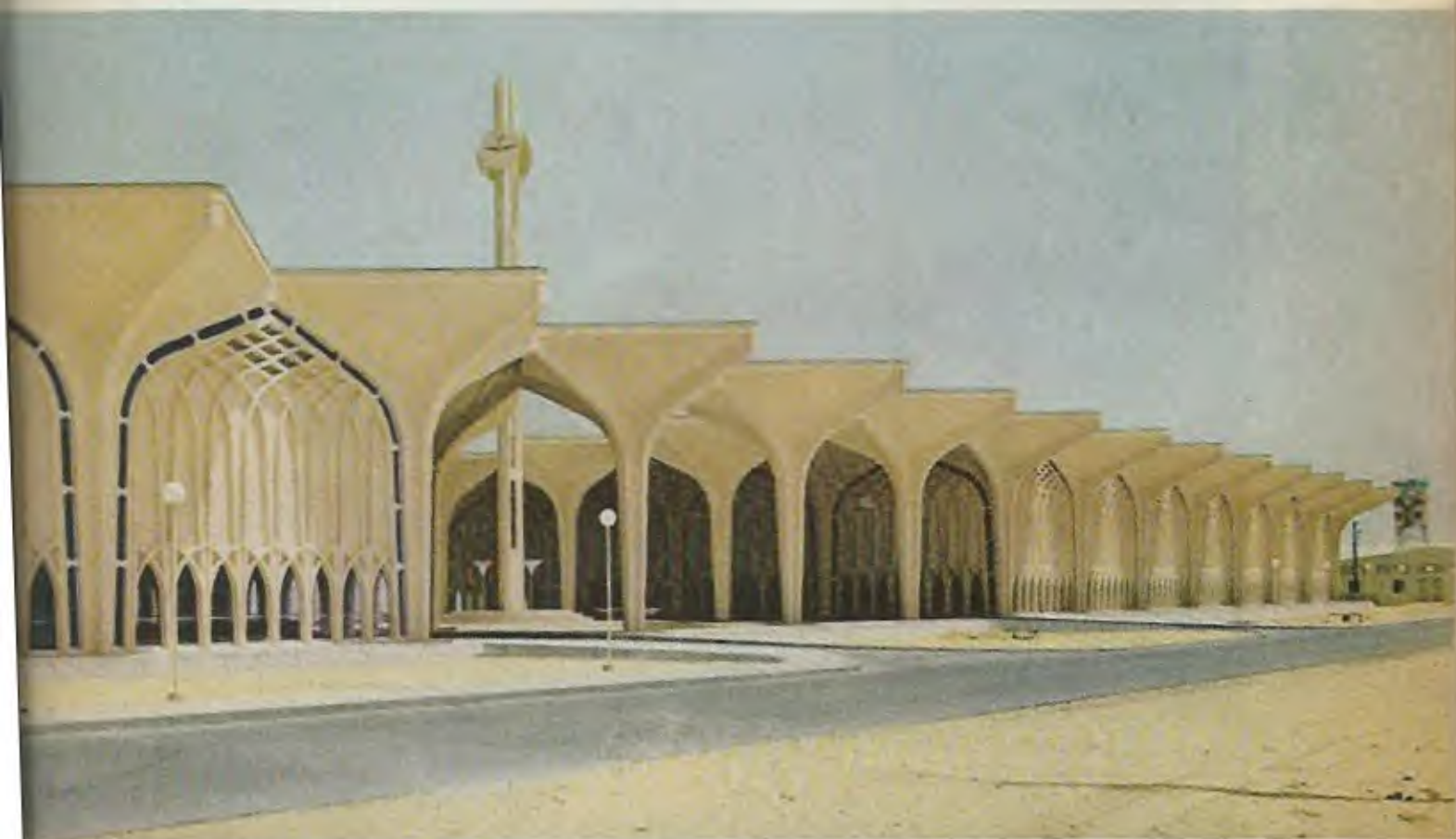
SAUDI ARABIA'S Civil Air Terminal at Dhahran was made "important and monumental," as befitting main gateway to
